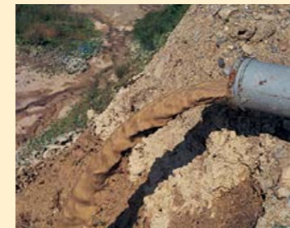
Removing slurry from a tunnel
