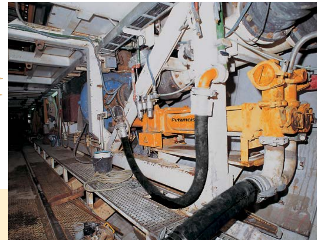
A KOV 1050 pumps the injection mortar behind the ring segment
