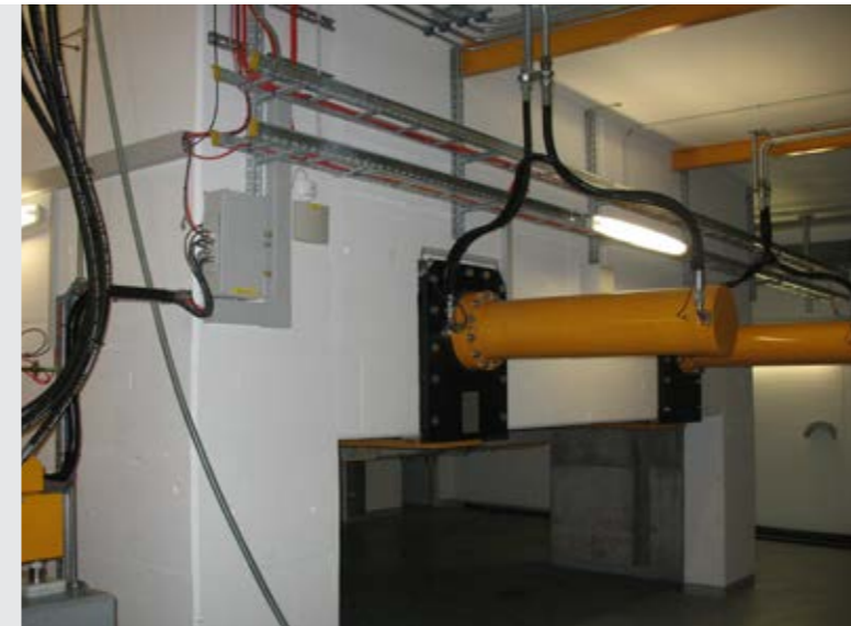
Sliding frame cylinder in a concrete silo, Sewage sludge plant Oftringen, Switzerland
