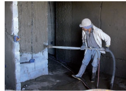
Spraying of plaster
