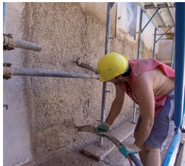
Spraying of exterior plaster
