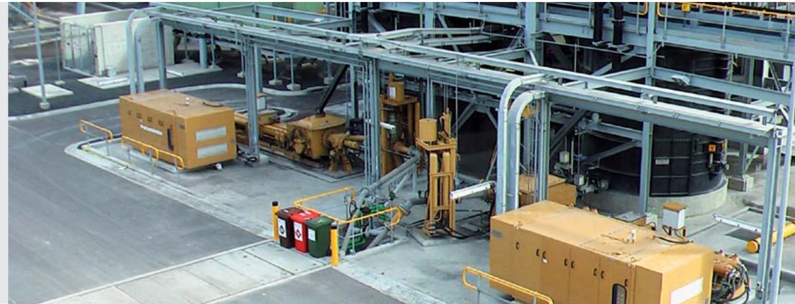
Redundant transport of fly and bottom ash from a power station
